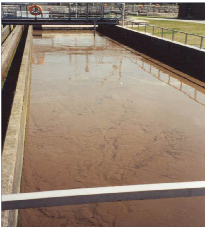
Fig. #43 - Poor mixing in long tank
