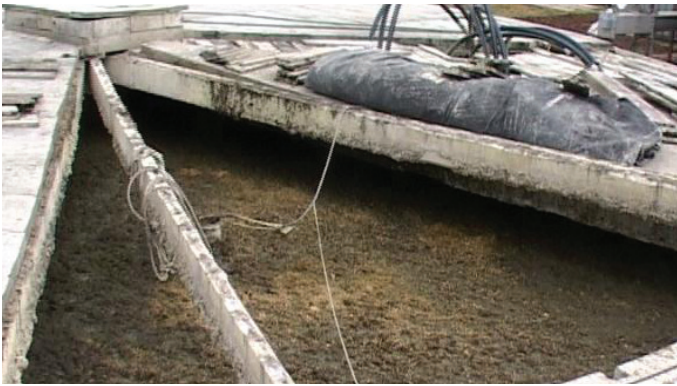
Fig. #10 - Anaerobic Digester Sludge - No Mixing
