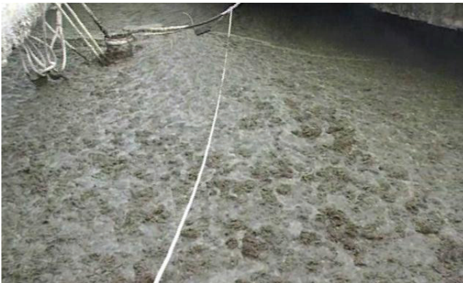
Fig. #11 - Anaerobic Digester Sludge - After Mixing
