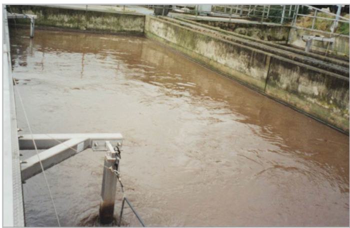
Fig. #44 - Good mixing in long tank
